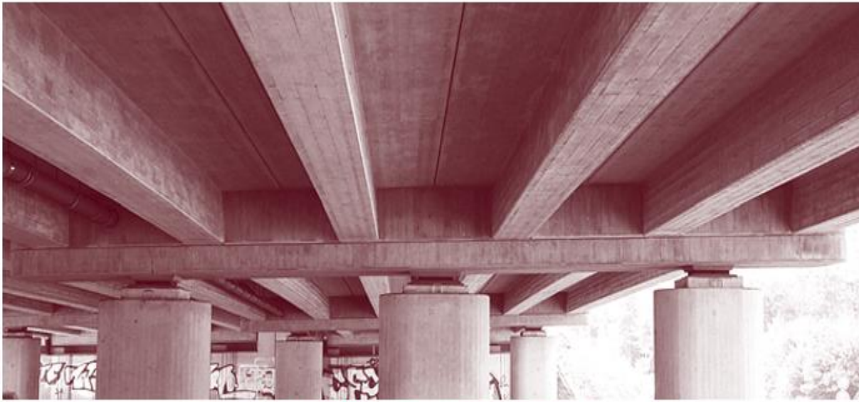
Figure 28. Precast, prestressed concrete bridge.
