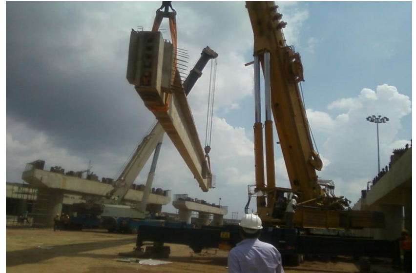
PROPER METHOD OF LIFTING HEAVY PRE CAST GIRDERS
