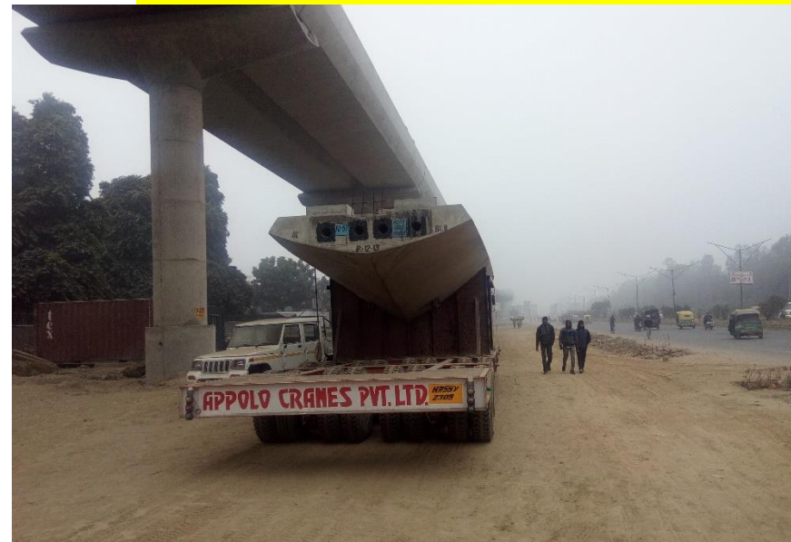
Transportation 80-90 ton Pier Head
