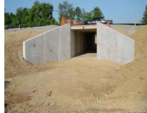
Pre cast Box Culverts with Pre cast Wing Walls
