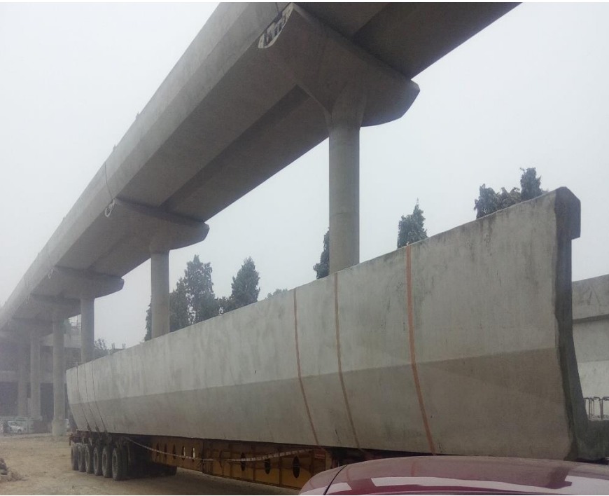
Transportation 180 ton Girder (Prestressed)- each side of Pier Head
