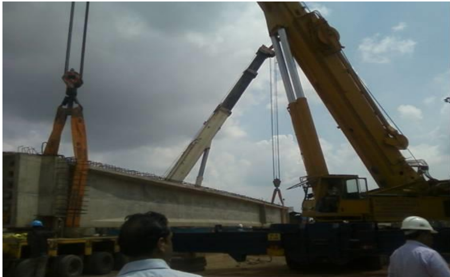
PROPER METHOD OF LIFTING HEAVY PRE CAST GIRDERS
