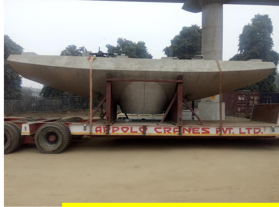
Transportation 80-90 ton Pier Head
